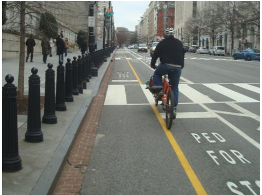
A two-way cycle track in Washington DC, in effect converting part of 15 th St. into a multi-use path..
