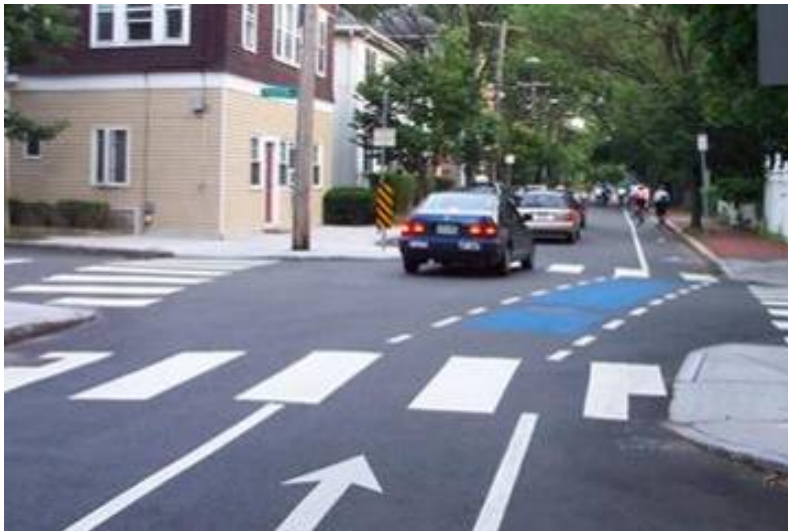
Coloring bike lanes – typically blue, as shown here in Cambridge MA – has emerged as a useful technique for guiding cyclists through complicated intersections.
