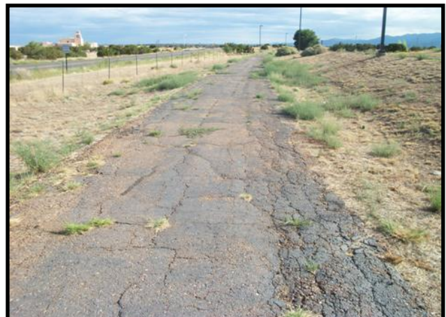
Deteriorating asphalt on the multi-use trail at the Santa Fe Community College. This trail was slated to be rebuilt by SFCC after this photo was taken in 2011.
