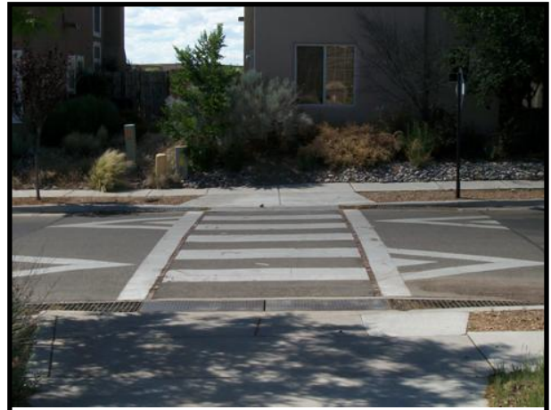
This marked crosswalk in Nava Ade incorporates a speed table to calm traffic where a trail meets a residential street.
