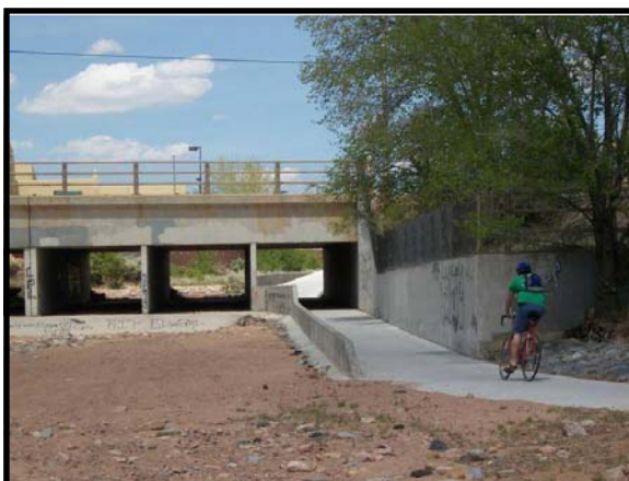
Retrofitting an existing culvert to create a trail underpass is a homegrown “best practice” that MPO members should seek to replicate elsewhere.
