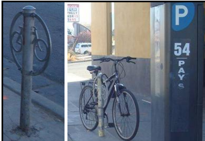
When pay stations replaced parking meters in Nob Hill, the City of Albuquerque converted the posts into attractive and functional pieces of the sidewalk streetscape.
