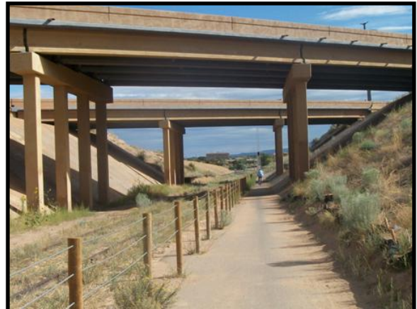
Grade-separated crossings of major roadways can be invaluable for trail users but are often prohibitively expensive unless integrated into an existing structure, such as the Santa Fe Southern Railroad's underpass of I-25.
