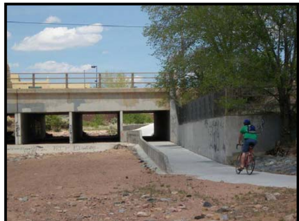
This grade-separated crossing of the Arroyo de los Chamisos Trail under Rodeo Rd. utilized an existing concrete box culvert, an achievement that is promoted as a “best practice” in Chapter VI.
