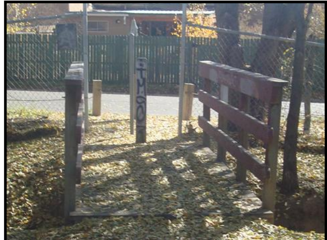
Existing bridges over the Acequia Madre include this two-by-four construction providing some degree of access between Otowi Rd. and Camino Canyon de Chelly (above). A similar construction (but without the center posts) could connect the Acequia Trail to the end of Kathryn St. (below)
