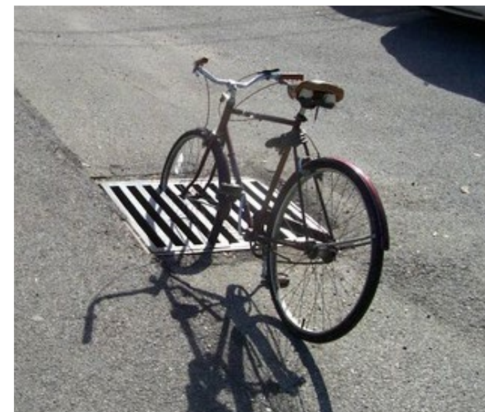
Unsafe Grate for Bicycles - Bike PGH
