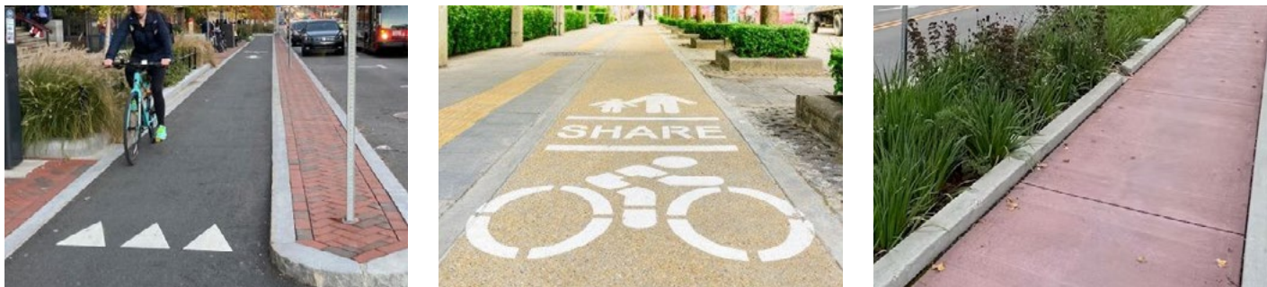
Surface treatments or paver materials that align with Santa Fe's style can be used for median-protected and raised bicycle facilities.
