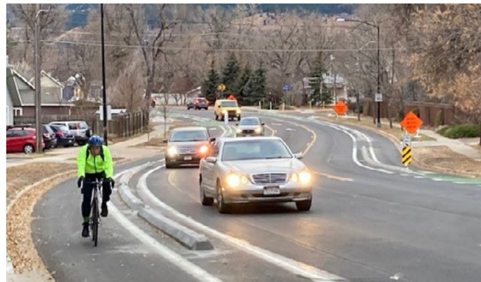
Curb separators on Folsom Street Boulder, CO.
