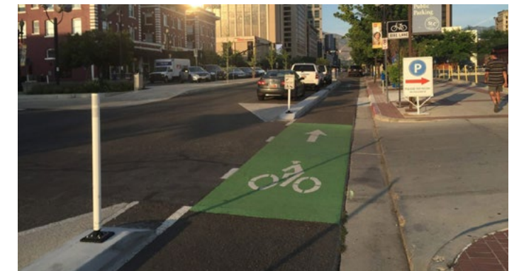
An example of green pavement used to highlight a bicycle facility at a driveway.
