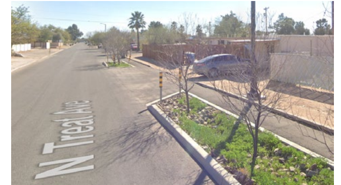
Bike facility improvements in Tucson utilizing raised medians and other measures to reduce conflicts at driveways and intersections.
