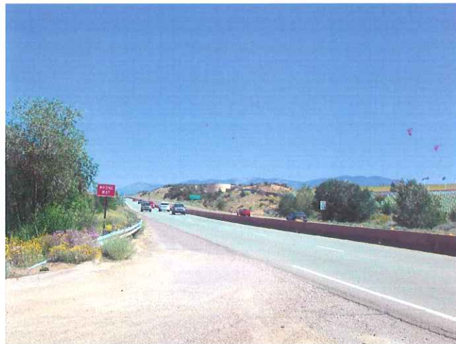
EB Viento Drive looking north onto St. Francis Dr.
