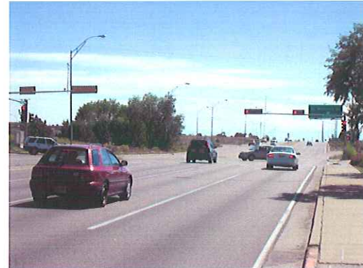
SB St. Francis at W. San Mateo Rd.
