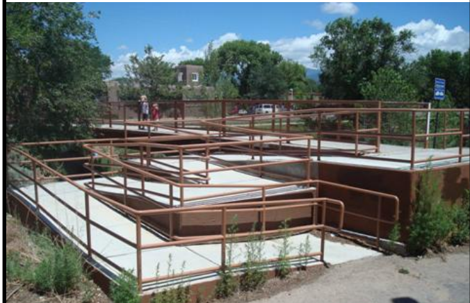
The two ends of the Closson St. footbridge across the Santa Fe River demonstrate how designs to provide access for wheelchair users can lead to contrasting outcomes for other users. The north side of the bridge (above) is well integrated into the narrow “River Trail” while the south side (below) is inaccessible for bicyclists and inconvenient for other users.
