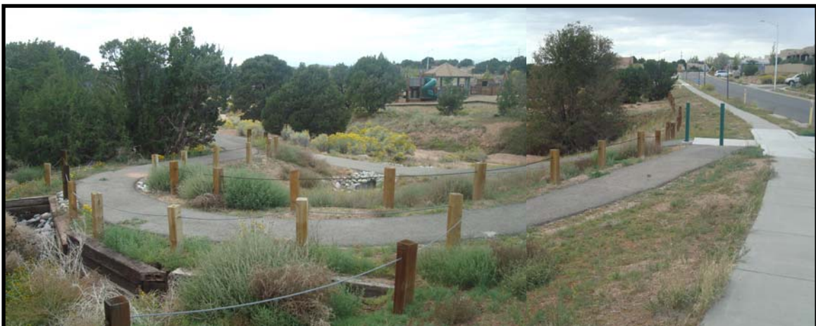
At another location in Pueblos del Sol where the existing trail was too steep to meet ADAAG grade requirements, a circuitous ADA-accessible route was created as an alternative, in foreground, while the more direct alignment was retained as the more convenient route for most users (background).
