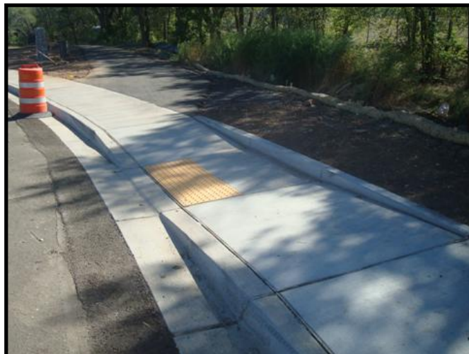
Acequia Trail at Potencia St.: NMDOT Standard Drawing meets ADA requirements but confines trail and sidewalk users to a narrow area along the edge of the roadway.
