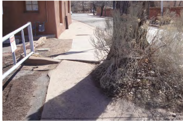
Cracked and buckled sidewalk
