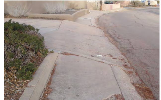
Steep curb cut for a driveway.
