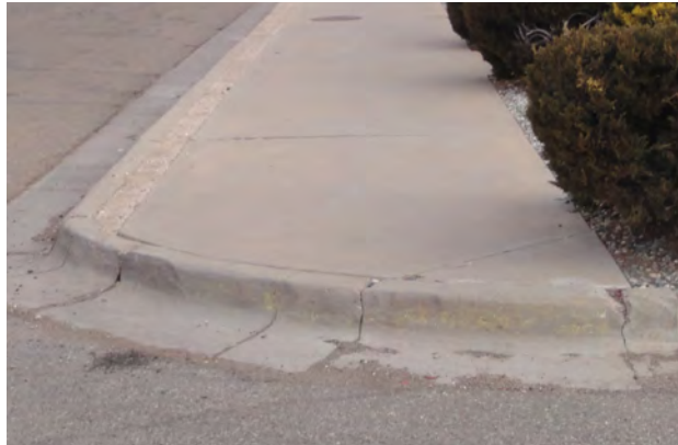
Tall sidewalk without a curb cut.
