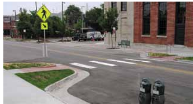
Figure 5.11: Bump-Outs Reduce Crossing Distance
