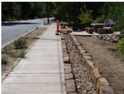
Storm water infiltration features that have been installed on Alameda Street
