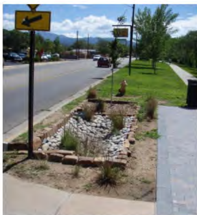
Storm water infiltration features that have been installed on Alameda Street
