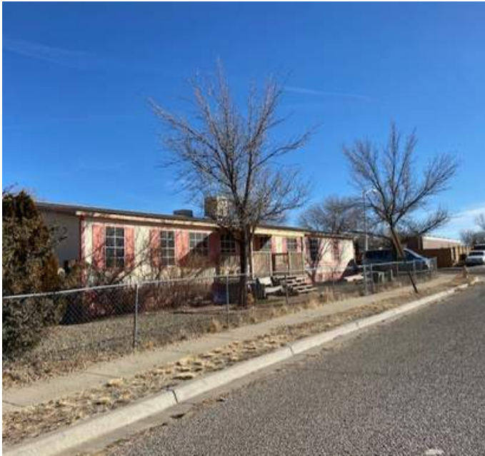
Image of mobile home in the study area Photo Credit: National Park Service (NPS), Rivers, Trails and Conservation Assistance program (RTCA)
