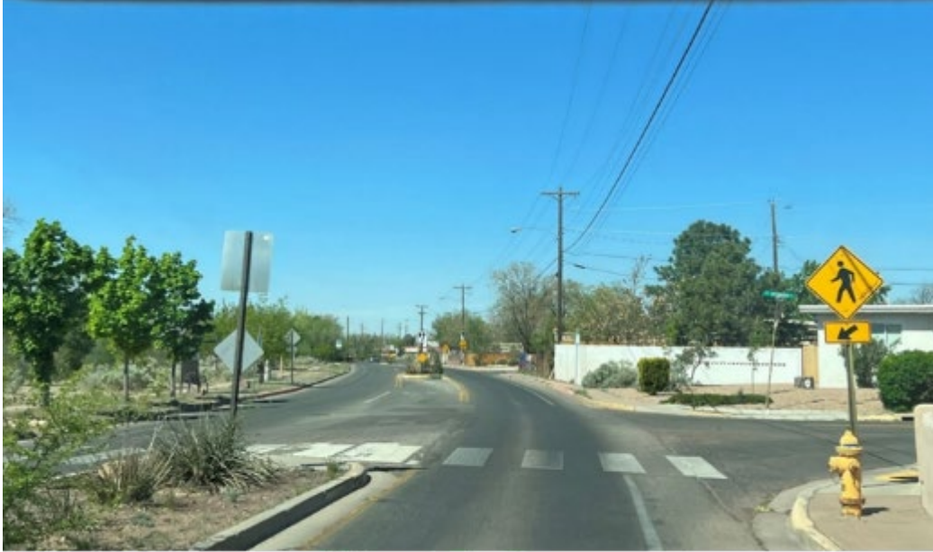
Figure 8. Photograph. Uncontrolled Pedestrian Crossing with marked crosswalk in City of Santa Fe (Source: FHWA).
