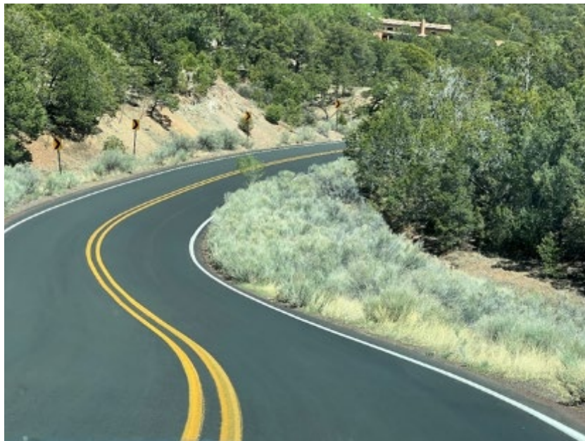
Figure 9. Photograph. Old Santa Fe Trail curves and chevron installation (Source: FHWA, 2022).
