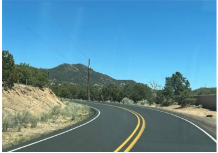
Figure 18. Photograph. Old Santa Fe Trail is a two-lane roadway that has rural design features and several curves along the corridor. Chevrons and advanced curve warning signs are not located on all curves with similar characteristics (Source: FHWA, 2022).
