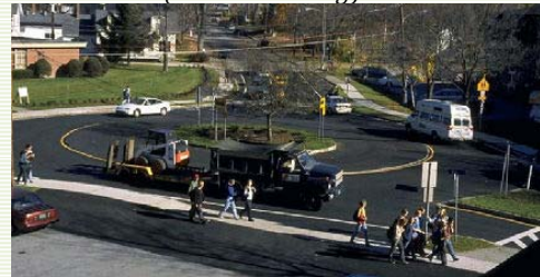
HAWK Pedestrian Signal (Saferoutesinfo.org)
