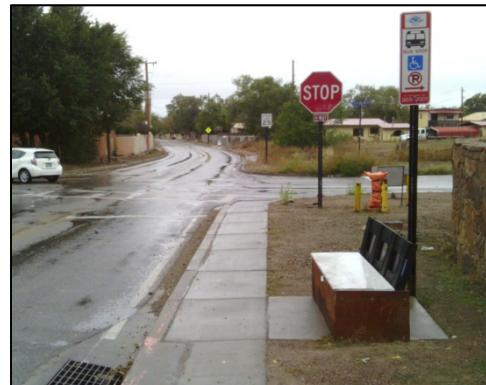
**Landing Pad Obstructed by Bench**
