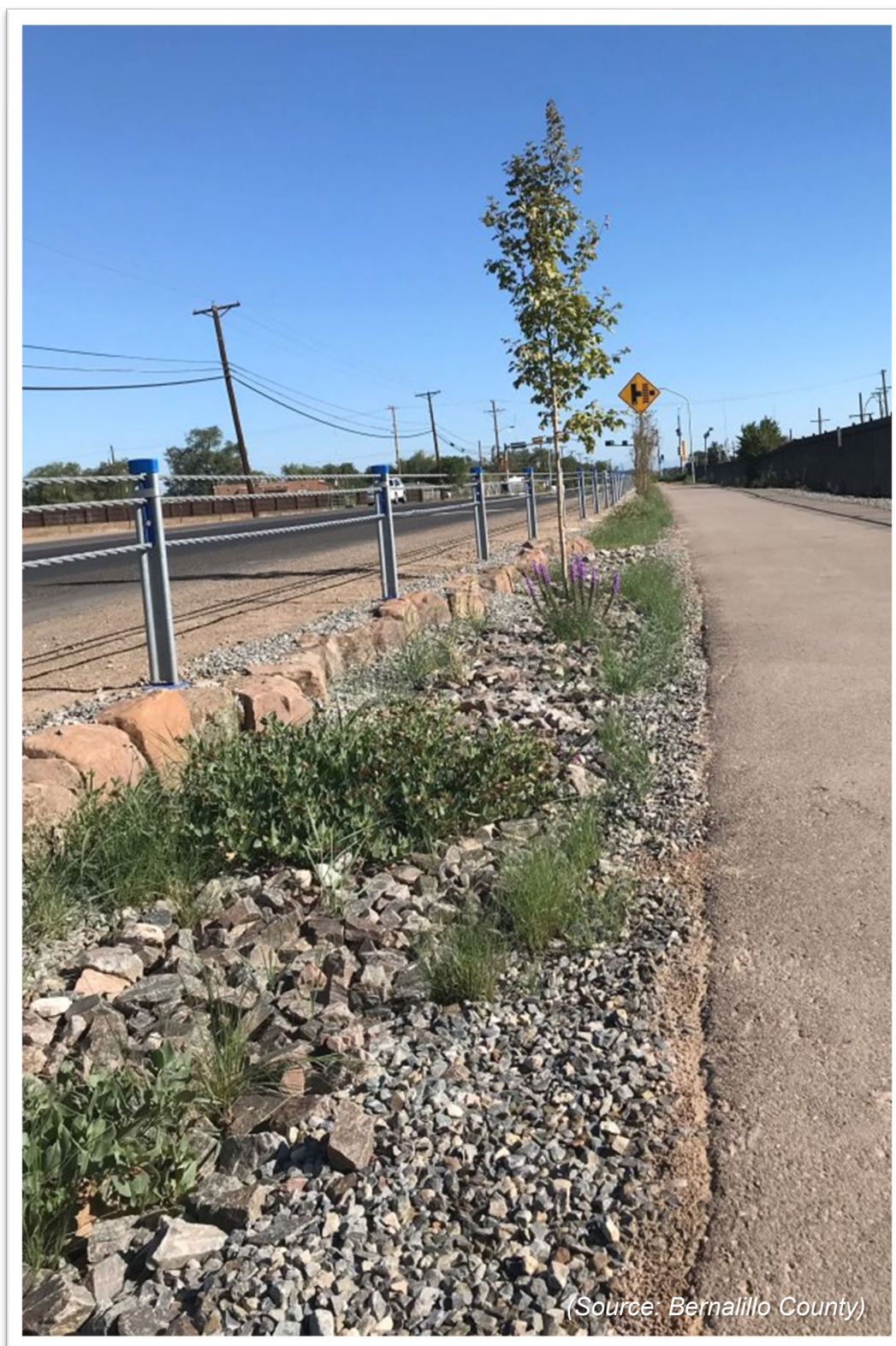
Figure 63: Bioretention Basin Constructed Along 2nd Street Trail
