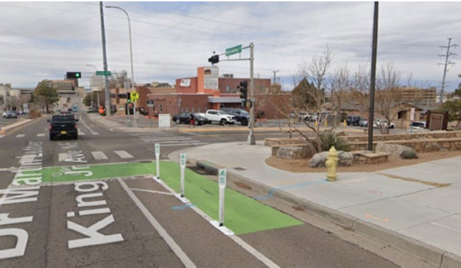
Protected bike facility in Albuquerque utilizing green paint and flexible bollards
