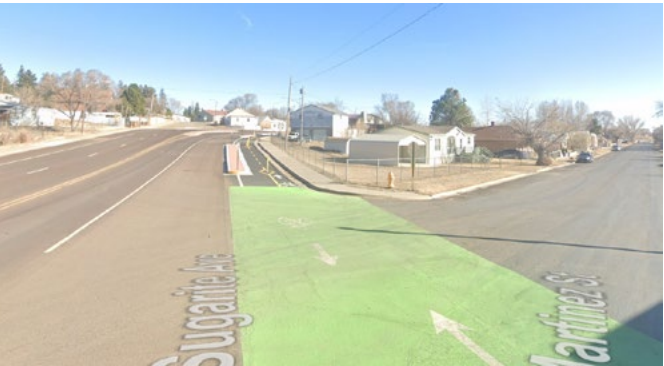
Protected bike facility in Raton utilizing green paint and raised medians.
