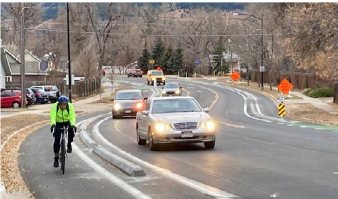
Curb separators on Folsom Street Boulder, CO.
