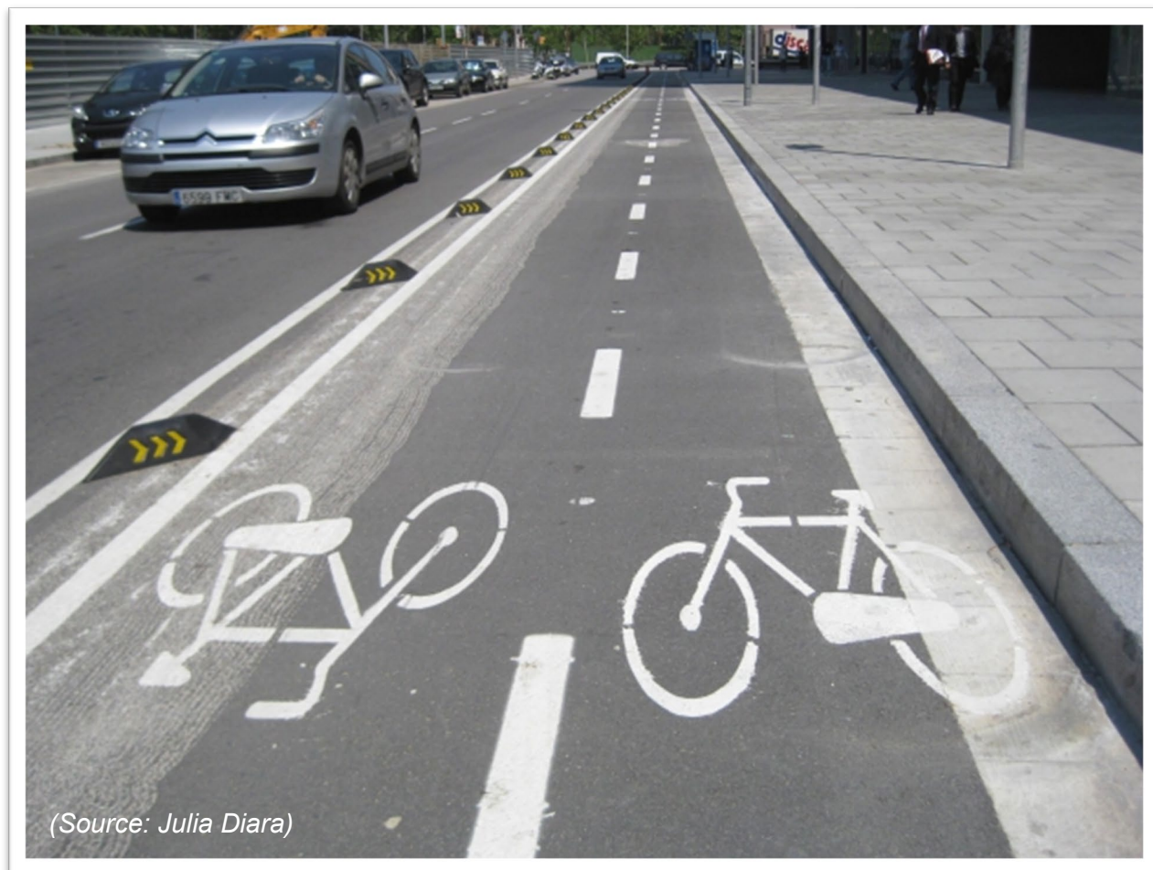
Figure 24: Rubber Barriers on a Two-Way Cycle Track
