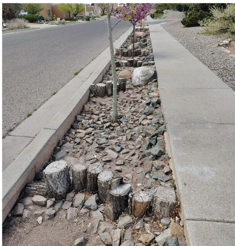
Figure 73: Check Dams Made from Wood
