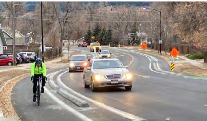
Curb separators on Folsom Street Boulder, CO.
