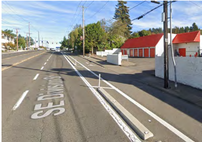
Protected bike facility in Portland utilizing green pain and curb stops.
