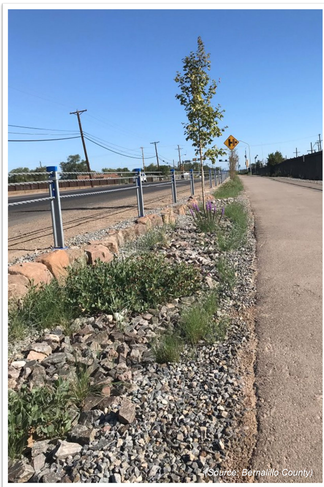
Figure 63: Bioretention Basin Constructed Along 2nd Street Trail
