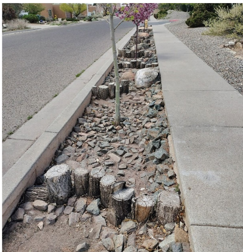
Figure 73: Check Dams Made from Wood
