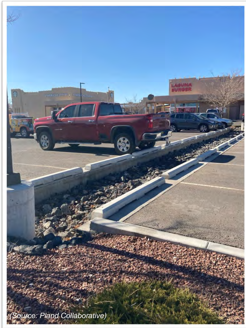
Figure 70: Infiltration trench in a commercial parking lot in Albuquerque, NM. This method can also be used along streets.
