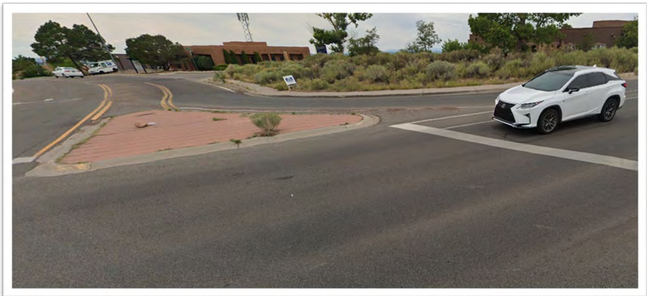
Figure 48: Mountable Curb Median Example
