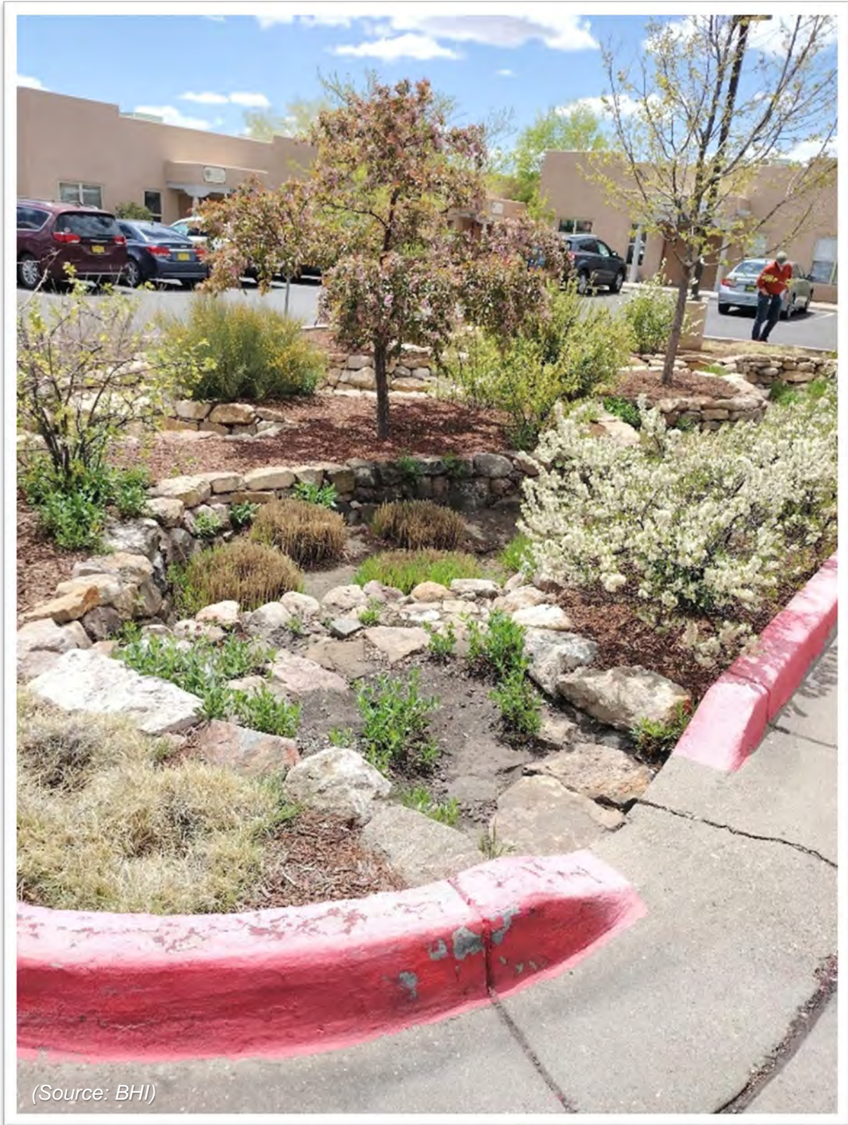
Figure 65: Bioretention Basin, also known as a Rain Garden, in Santa Fe. Note Rock Sediment Trap at Curb Opening
