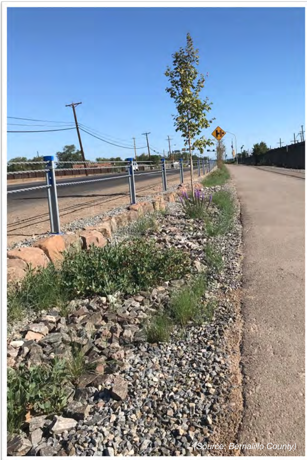
Figure 63: Bioretention Basin Constructed Along 2nd Street Trail
