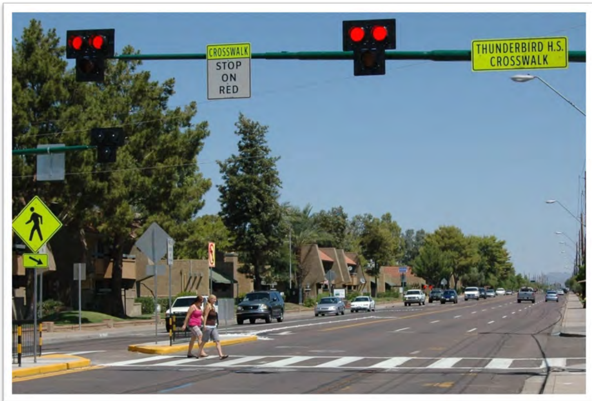
Figure 41: HAWK Beacon and Crossing
