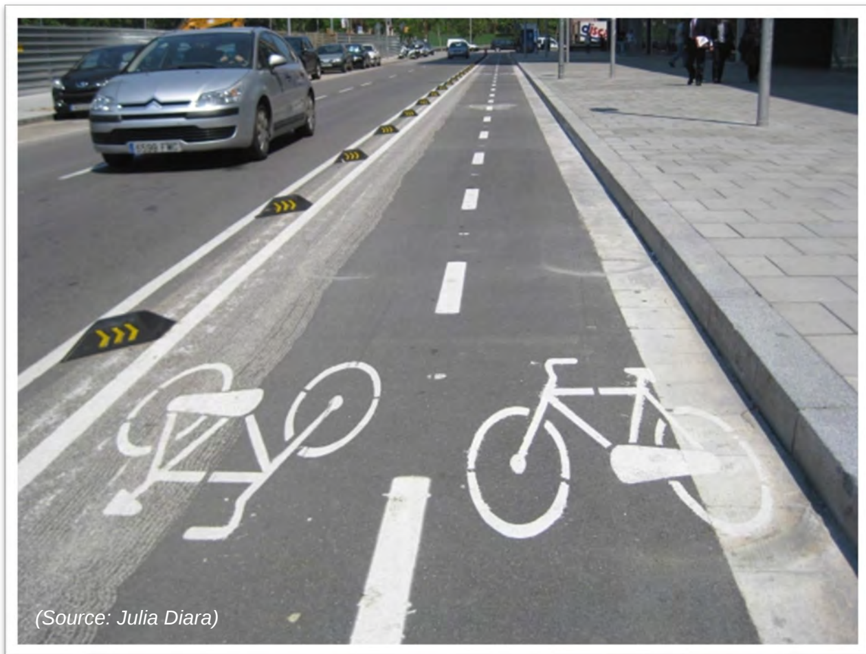
Figure 24: Rubber Barriers on a Two-Way Cycle Track
