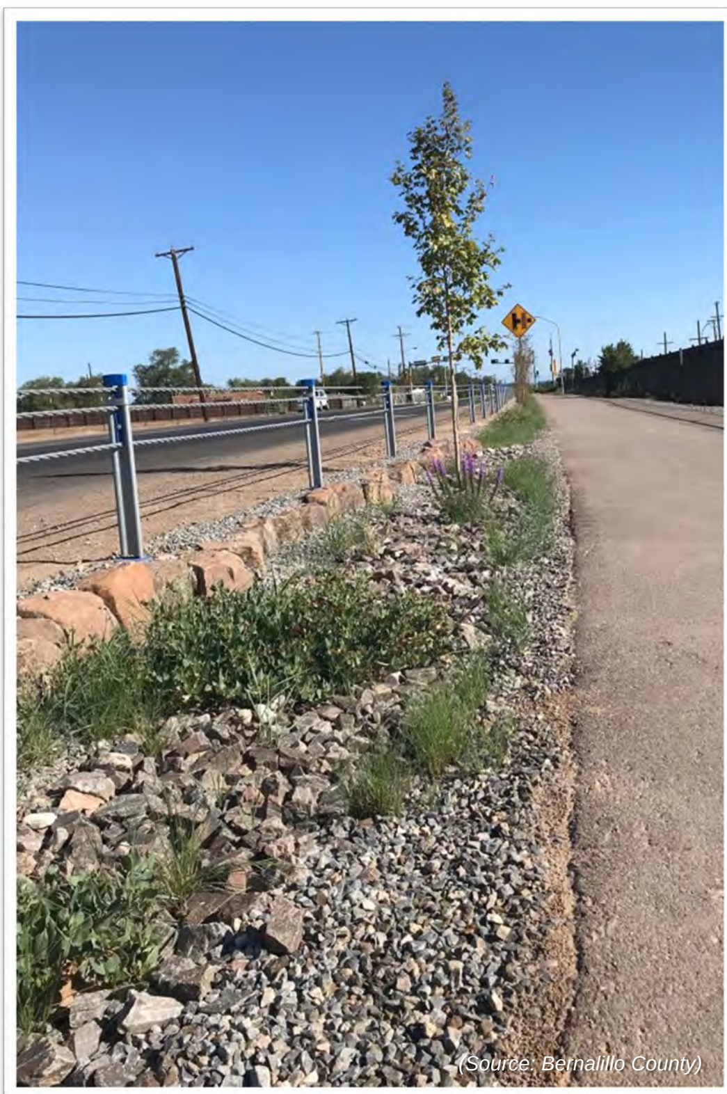
Figure 63: Bioretention Basin Constructed Along 2nd Street Trail, Bernalillo County, NM
