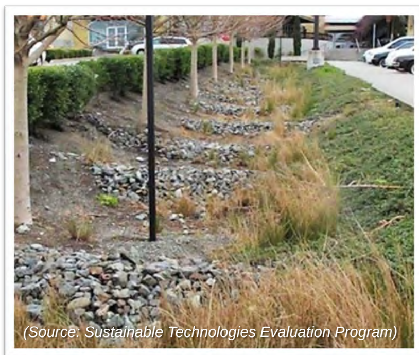
Figure 72: Check Dams Made with Rock
