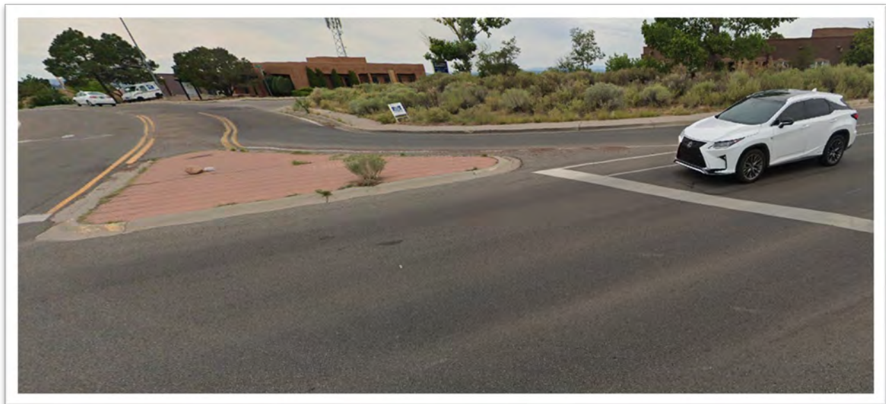
Figure 48: Mountable Curb Median Example
