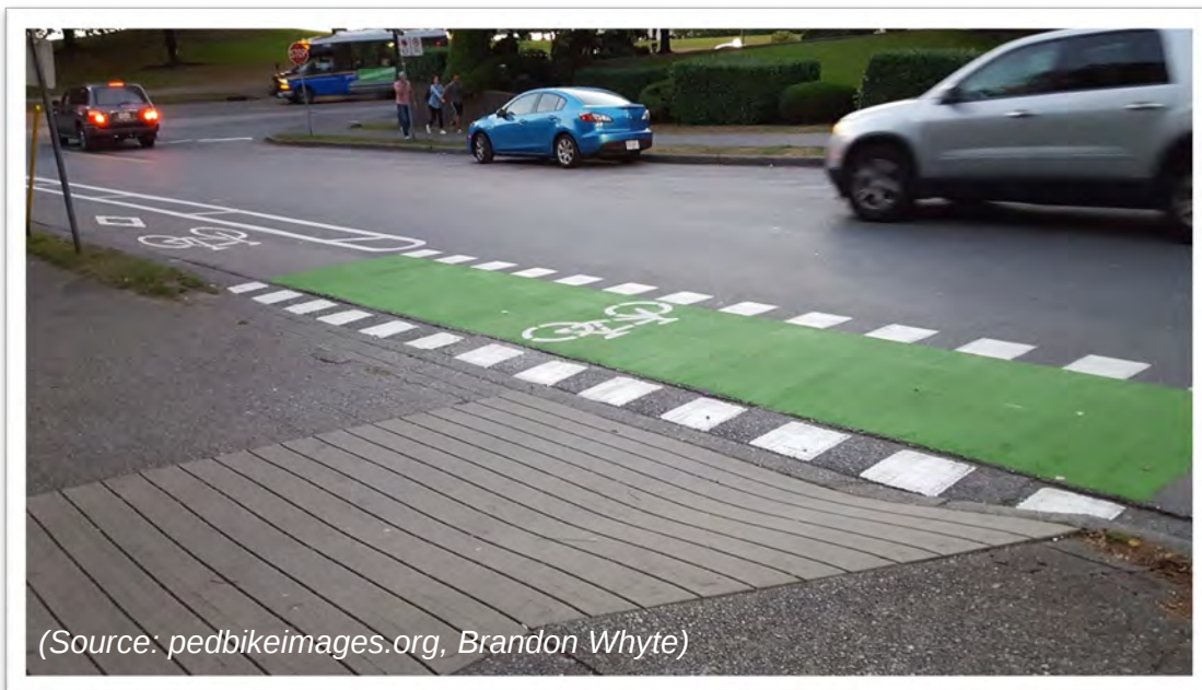
Figure 22: Raised Bike Lane
