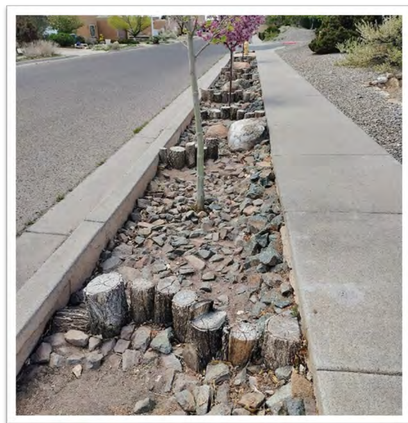
Figure 73: Check Dams Made from Wood
